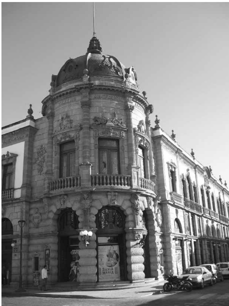
Figure 2 – Macedonio Alcalá Theatre in Oaxaca is an illustrative example of early 20 th century architecture with metallic structural and ornamental elements.
