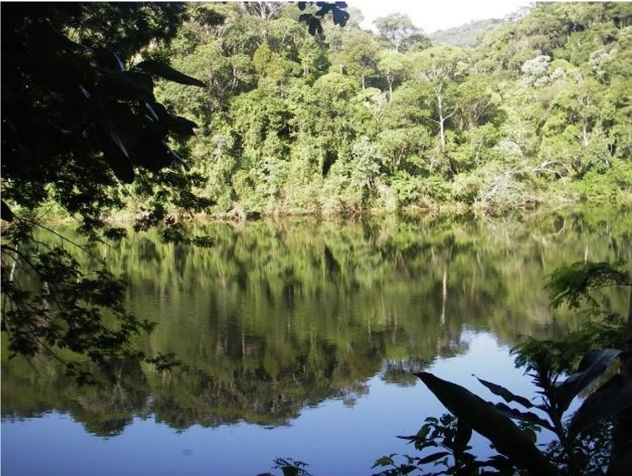
Figure 2 Camorim dam, seen from the retaining wall: water mirror and forest.
