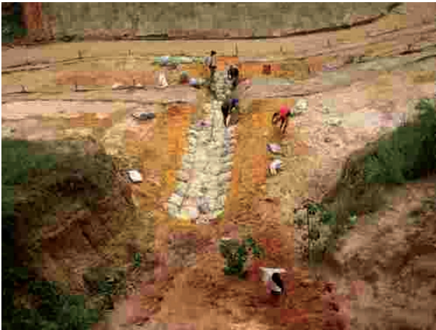
Figure 6 Gullied area in São Luis Municipality, Maranhão State, during rehabilitation work .Photo by Jose Fernando Rodrigues Bezerra.
