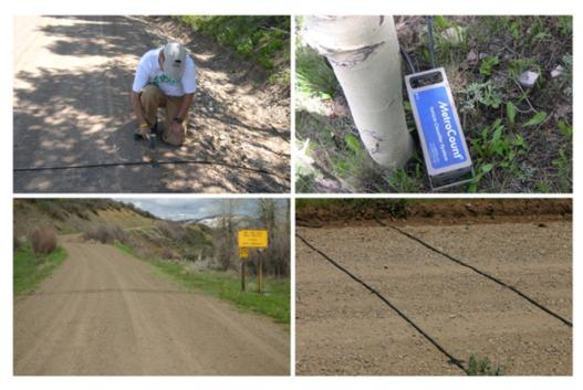
Figure 2. Images of a pneumatic counter, clockwise from top left: author installing pneumatic tube on the road surface; battery-powered electronic monitoring device; parallel pneumatic tubes across the road; typical view of a pneumatic counter across a road in the study area.
