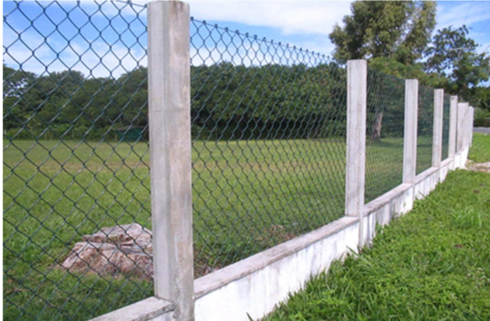
Figure 1. An example of the 1.5m high chain-link capybara fence evaluated for the cost-benefit analyses (Copyright © 2011, by Manetoni). Note that the fence in the photo shows a concrete bottom/foundation. For our cost-benefit analyses we did not include this concrete foundation; instead the chain-link fence extended to the ground.
