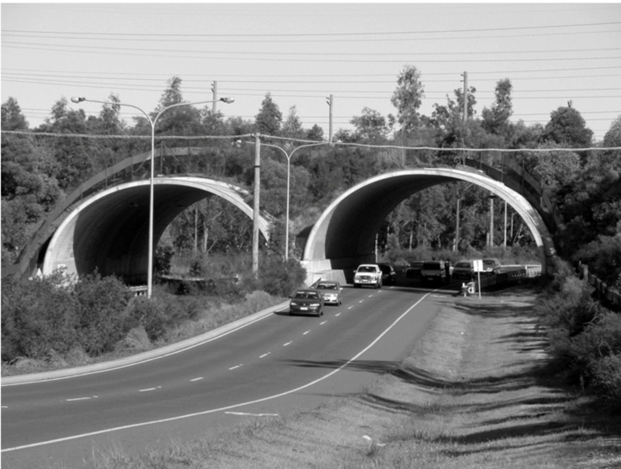
Figure 1. The Compton Road fauna overpass showing vegetation as developed about five years after construction.
